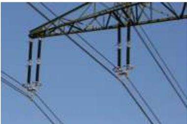
Figure 3 – Insulator on a high voltage power line separating the cable from the pylon. From [http://commons.wikimedia.org/wiki/File:Infrared\\_1080967.jpg](http://commons.wikimedia.org/wiki/File:Infrared_1080967.jpg)
