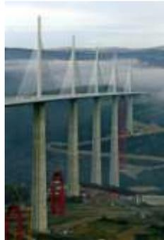
*Millau Viaduct constructed from concrete and steel because of their mechanical properties*
