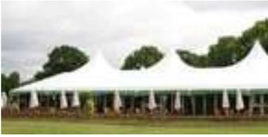
Marquee roof made from reinforced PVC fabric.
