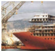
Welded sub-assembly being added to the hull of the passenger ship Seven Seas Navigator (Courtesy: Hydro Aluminium)
