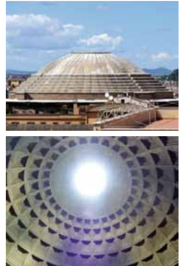
Figure 2 – The concrete dome of the Pantheon in Rome showing the exterior (top) and interior (bottom). ( http://en.wikipedia.org/wiki/File:Pantheon_dome.jpg and http://upload.wikimedia.org/wikipedia/commons/8/88/Pantheon_chiesa%2C_Roma_fc07.jpg )
