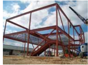
Figure 14 – Mild steel used in the construction of buildings. ( http://www.davisiron.com/graphics/Texas_Land_Bank.jpg )
