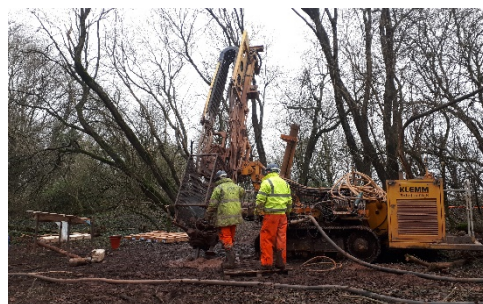
Inclined core drilling (generic example)
